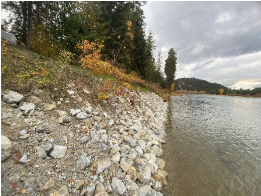
Completed and planted McGuire Project
